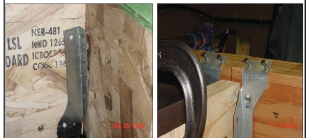
Face Mount failure
