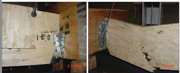
Nail withdrawal / overturning failure
